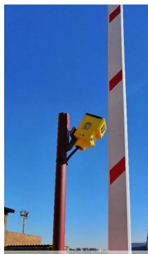
Proximity beams are used to keep the boom open while truck moves on and off the bridge.
